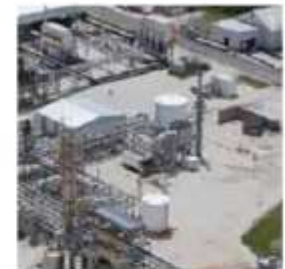
Step 6: Renewable power generation
