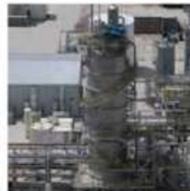
Step 4: Fermentation (bioethanol production from syngas through biological process)
