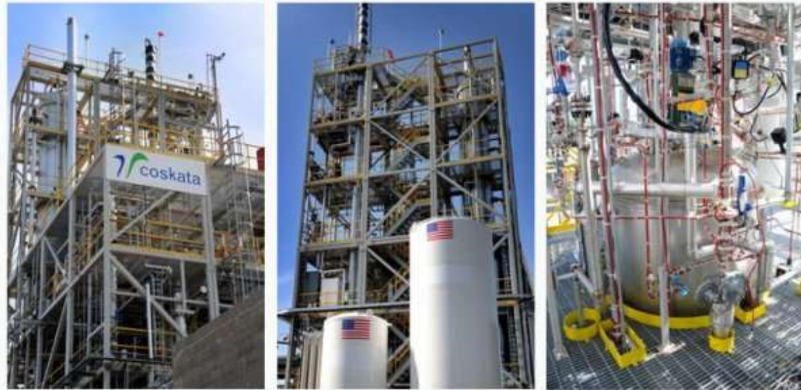
Coskata's semi-commercial FlexEthanol™ facility
